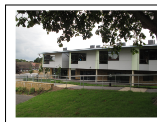
Balfour extension completed in 2009
