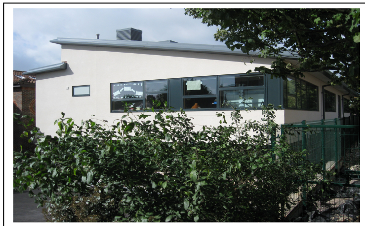
Davigdor Extension completed 2010
