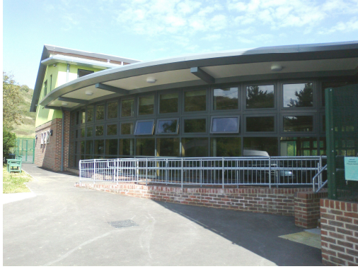
Whitehawk extension completed 2011
